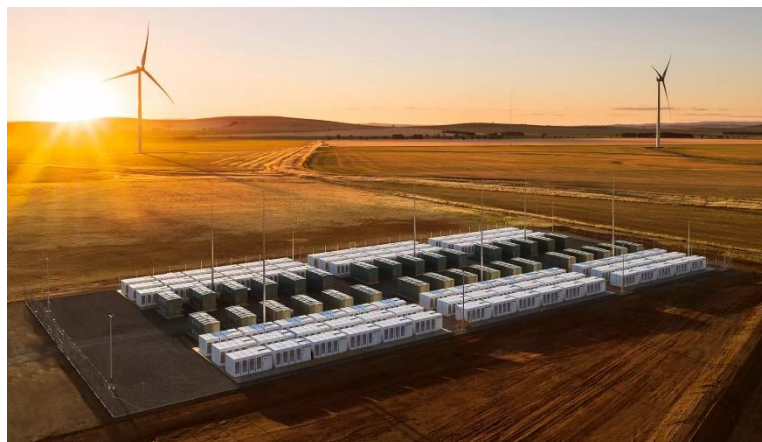
Figure 58: Tesla 50 kW/ 201 kWh Powerpack-based energy storage system adjacent to the 315 MW wind farm of the Hornsdale Power Reserve, in Australia, owned and operated by French company Neoen. Picture obtained from 127 .
